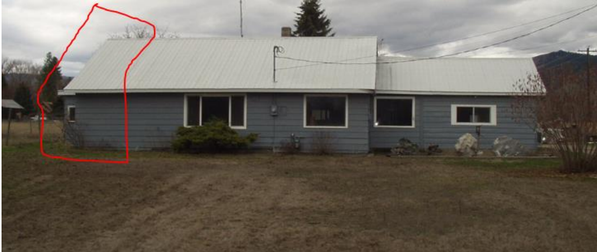
Figure 5: Roof Sagging at Southeast Corner of House (Looking West)
