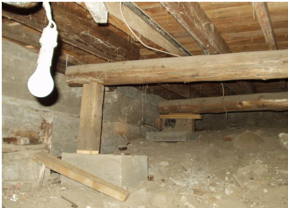
Figure 2: North Crawlspace Foundation Wall (Soil Eroded) and Typical Floor Framing (Looking East)
